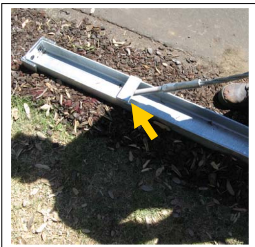
Figure 19. Push cables under steel strap on Ground Strut.
