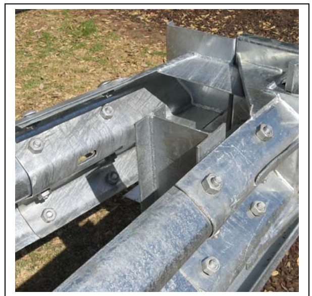
Figure 46. Use 8 standard splice bolts.
