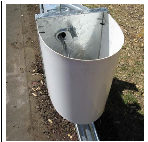
Figure 27. Attach nose using nylon push rivets.
