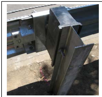
Figure 15. Bolt rail 1 and blockout to post 2.
