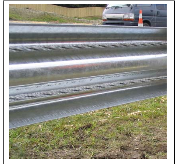
Figure 26. Tighten cables until they are taut.
