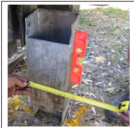
Figure 4. Measure 8 in. towards roadway.
