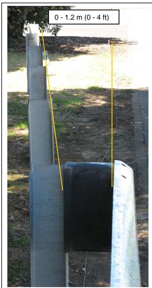
Figure 29. Pull string line to follow roadside edge of posts.
