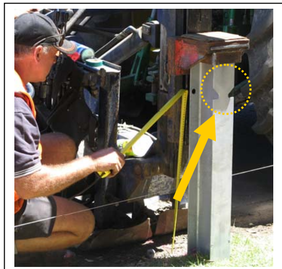
Figure 2. Notches go to the backside.
