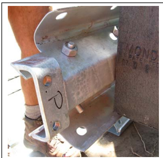
Figure 10. Bolt Slider Bracket to end of rail 2 at post 3.
