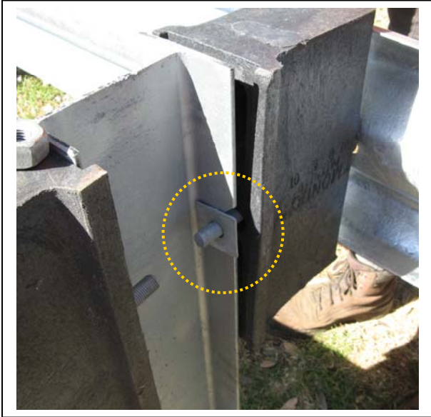
Figure 43. Bolt rail 1 and blockout to post 2 using the square washer.
