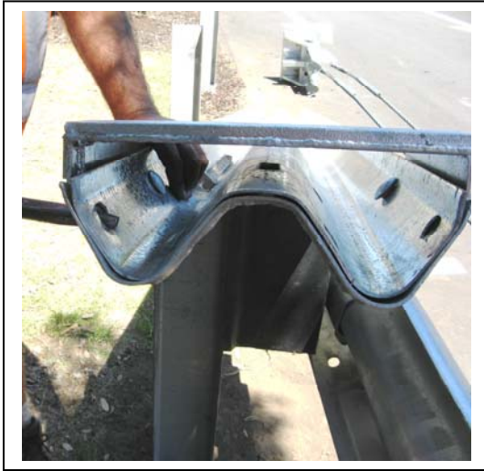
Figure 12. Sit rail 1 so it is raised off the ground.
