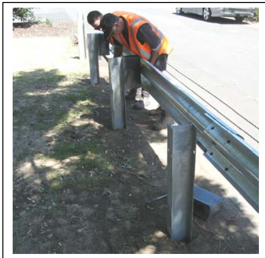
Figure 8. Bolt rail 2 to post and blockouts.
