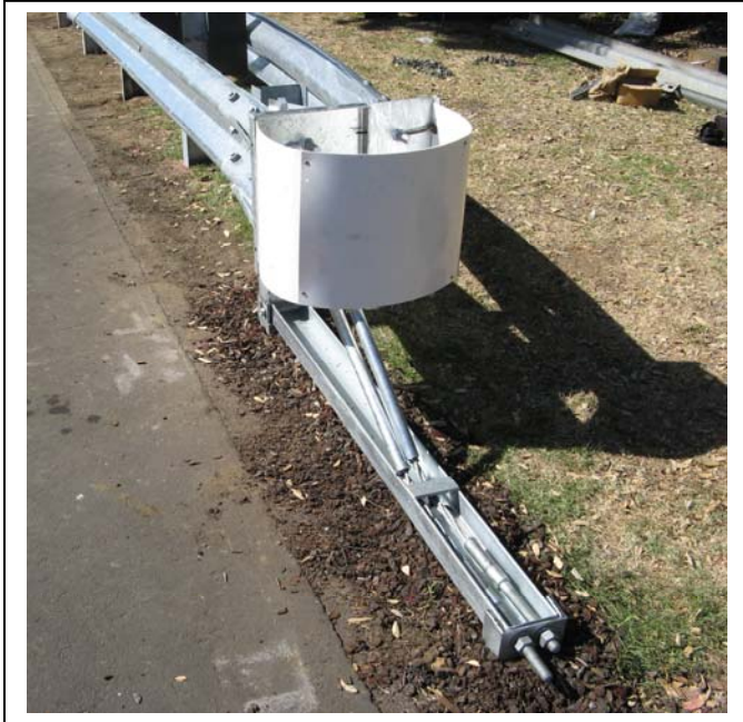
Figure 47. Attach nosing using nylon push rivets.
