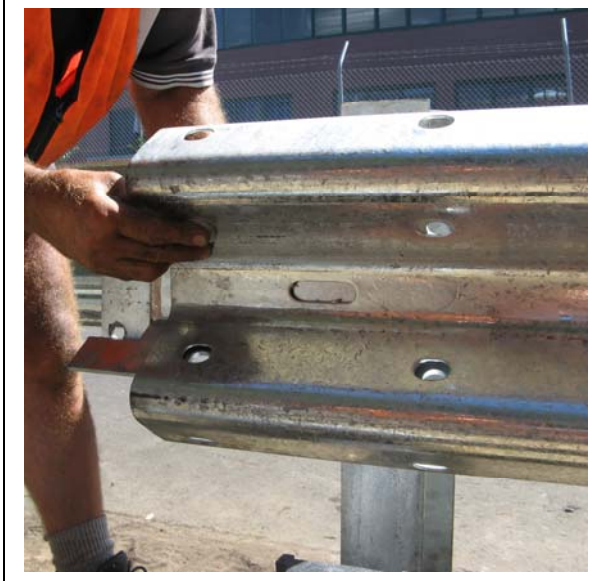
Figure 39. Bolt Slider Bracket to upstream end of rail 2.
