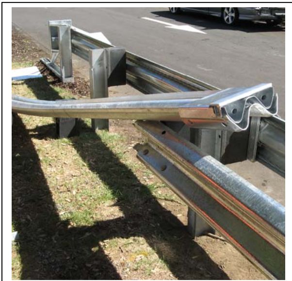
Figure 41. Fit the Slider Panel onto the straight end of rail.
