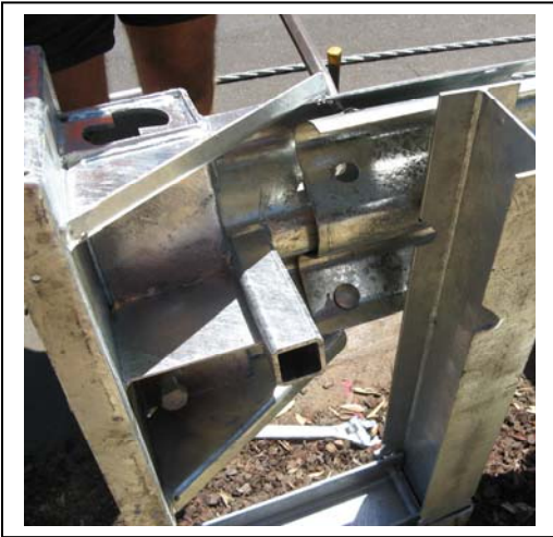
Figure 17. Attach Impact Head to rail 1.
