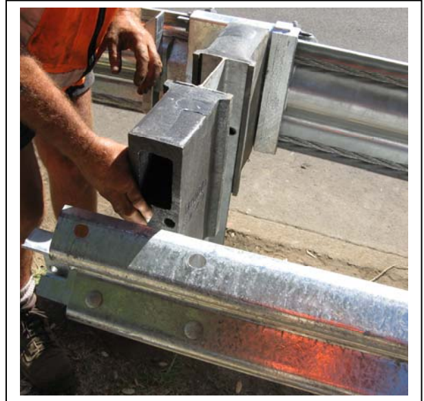
Figure 40. Angle bar end should be closest to Impact Head.
