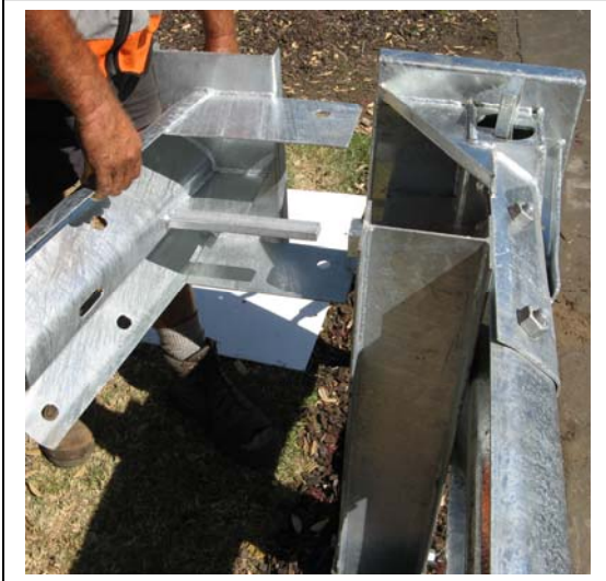
Figure 35. Fit secondary head to main head.
