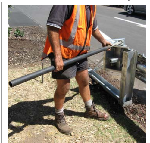
Figure 23. Use crow bar to turn Friction Plate.
