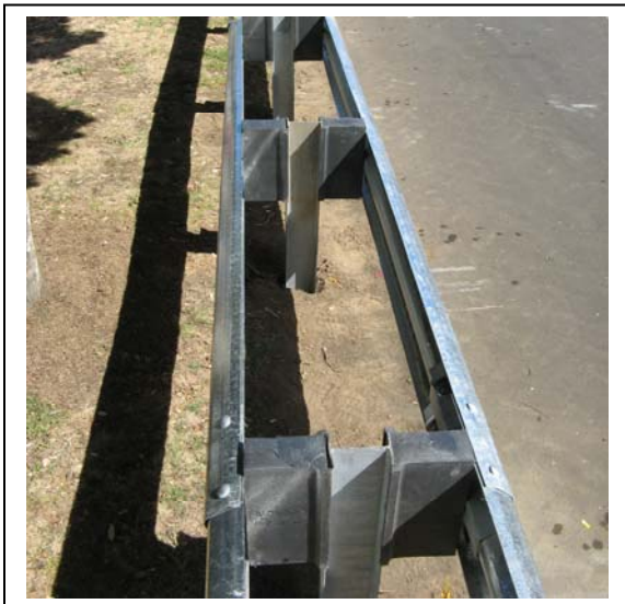
Figure 37. Rails installed with blockouts.
