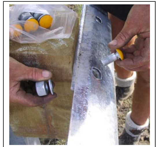
Figure 9. Splice rail 2 to rail 3 with 8 special shear bolts.
