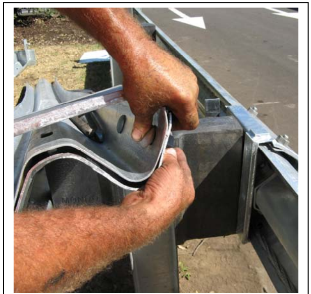
Figure 42. Push bolt from inside (nut on traffic face).
