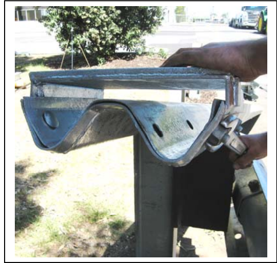
Figure 13. Slide the Slider Panel onto downstream end.
