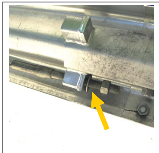
Figure 22. Do not tighten nuts at this time.
