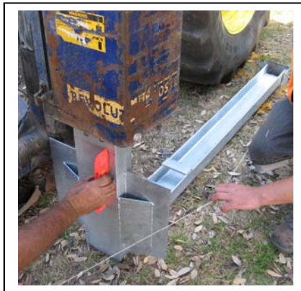
Figure 5. Drive post 1 into augured hole.
