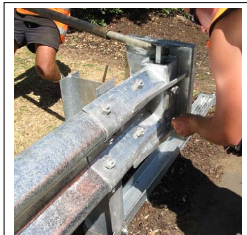
Figure 24. Use socket to lock bar in the turned position.
