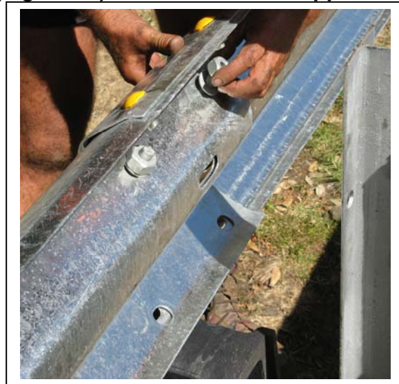
Figure 38. Splice rail 2 to rail 3 with 8 special shear bolts.
