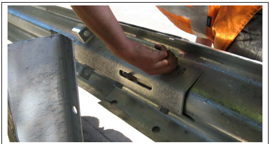
Figure 7. Splice rail 3 to rail 4 with 8 standard splice bolts.
