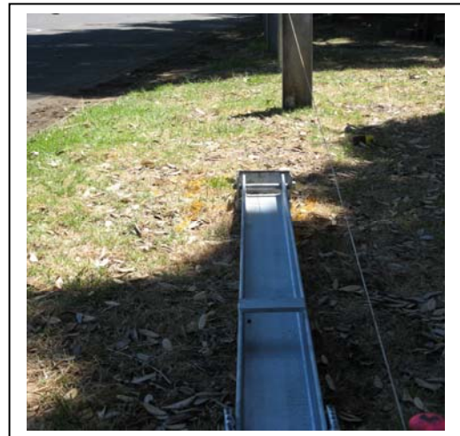
Figure 31. Place Ground Strut parallel to string line.
