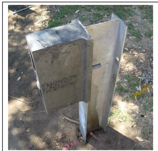
Figure 3. Bolt the blackout prior to attaching the rail.
