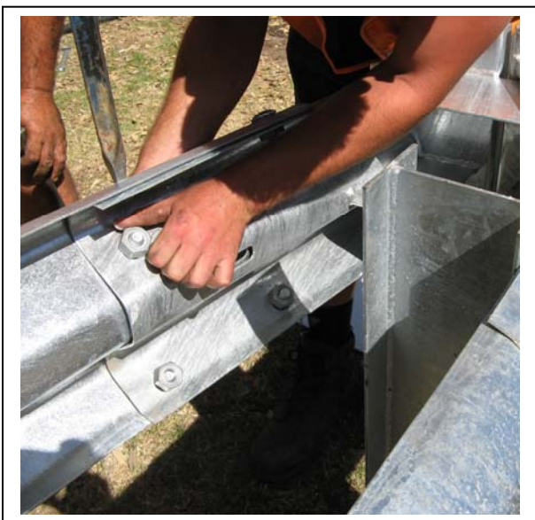
Figure 45. Splice the rail to secondary impact head.
