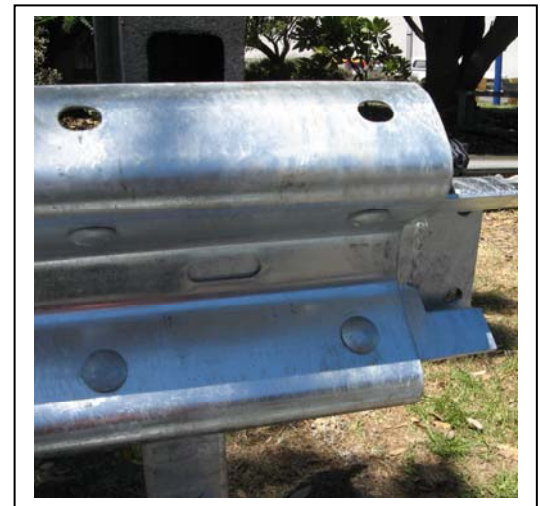
Figure 11. Remove angle bar bolts.
