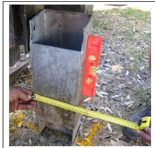
Figure 30. Place roadside face of post 1 towards roadway.
