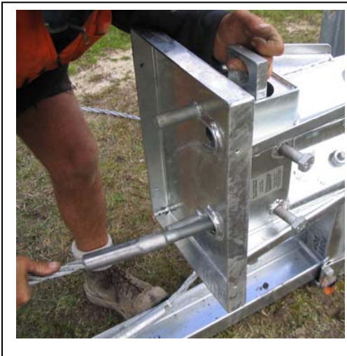
Figure 21. Pass the cable through the bottom hole.
