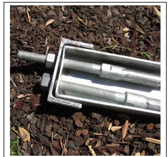
Figure 20. Thread the nuts as shown.
