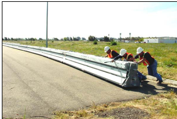
Figure 18. To deploy a barrier wall that is stored against a curb, move the end of the barrier out so that the truck can gain access.
