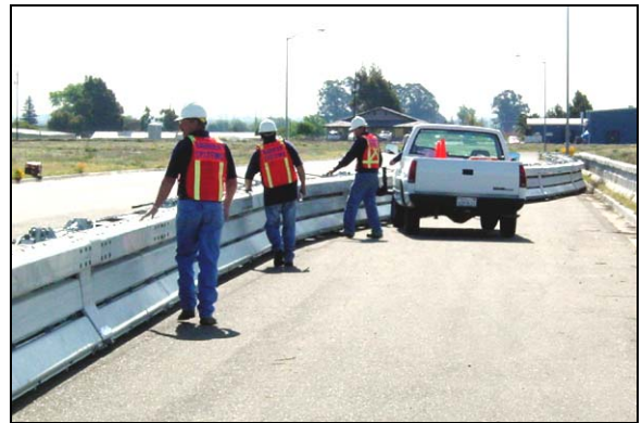
Figure 20. As the wall is being repositioned personnel lower each section at its final deployment or storage position.
