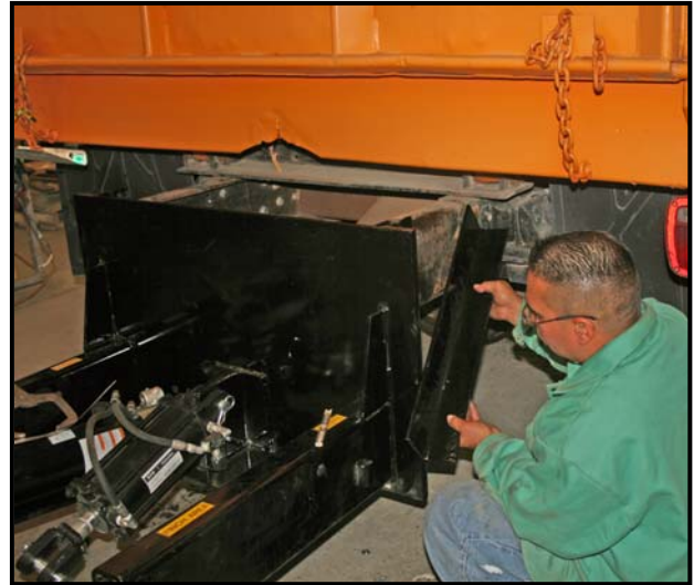
Figure 7. Install side Channel Braces.
