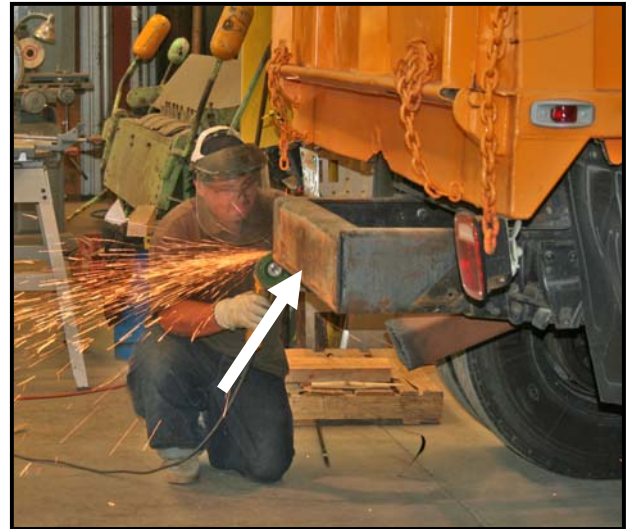
Figure 2. Connect the ends of the rails.
