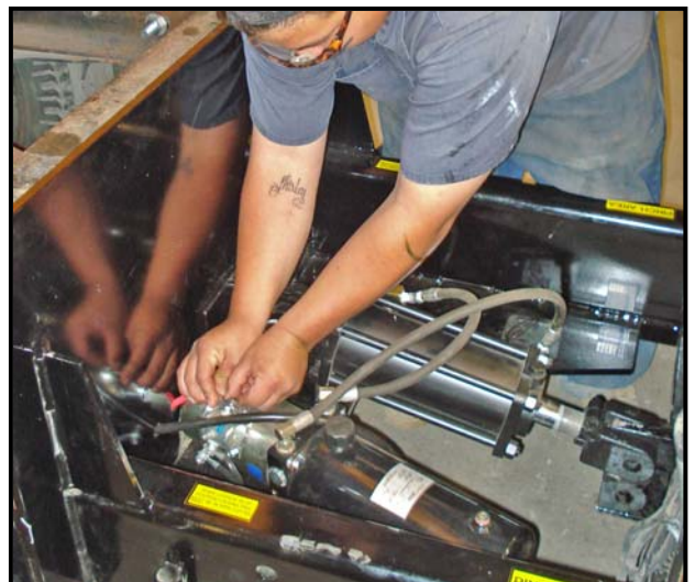
Figure 14. Attached to Support Structure.
