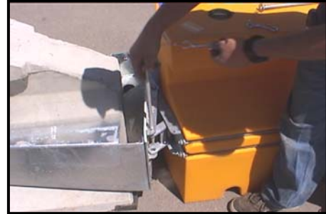
Install the pin with clip
