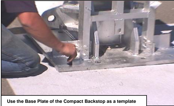
Use the Base Plate of the Compact Backstop as a template
